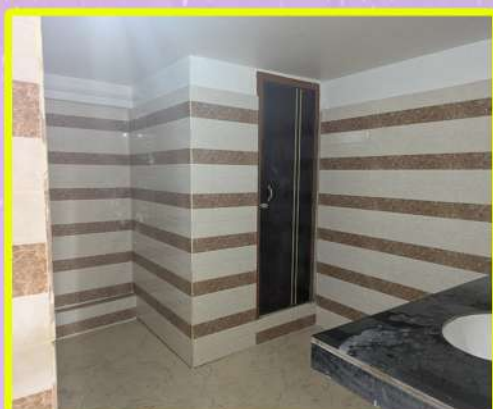
NEWLY RENOVATED BOYS' WASHROOM
